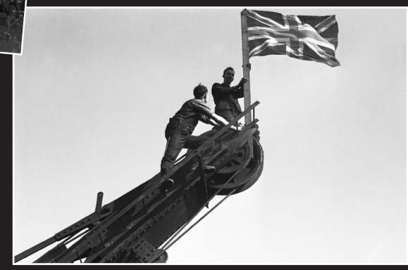
Two daring men raise the victory flag on the top of a crane in 1945. Health and safety had not been invented then!
