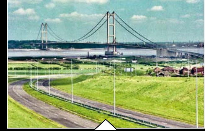
The almost completed Humber Bridge in March 1981. The approach road is finished but the embankment is without the modern day tree covering
