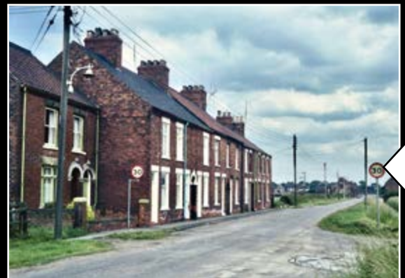
This row of houses on Far Ings Road, was demolished to make way for the approach road.
