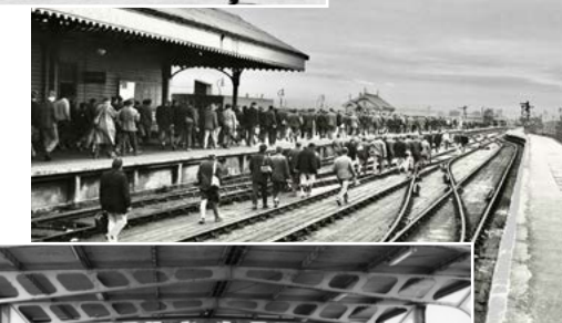
Workmen rushing to catch buses to a South bank construction project in 1969.
