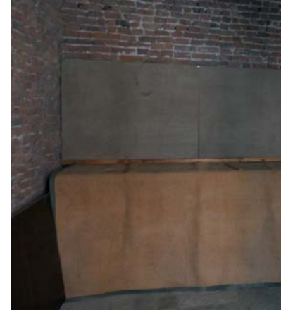
Stable Block interior
